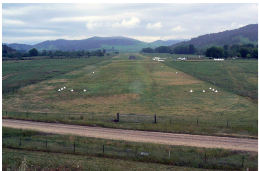
A view from the top of the dam wall looking north along RWY 31.
