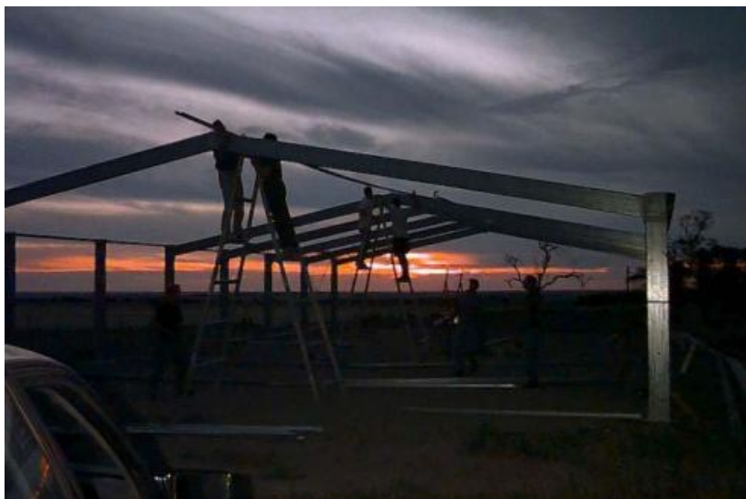
Left: The original hanger build at Lochiel.
