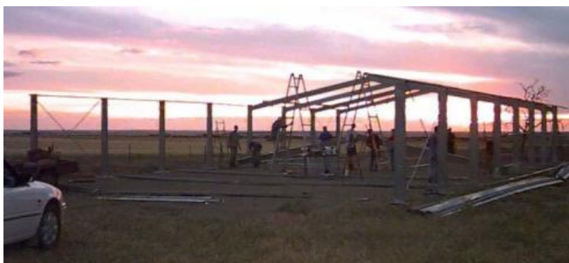
Below: The original hanger takes shape.
