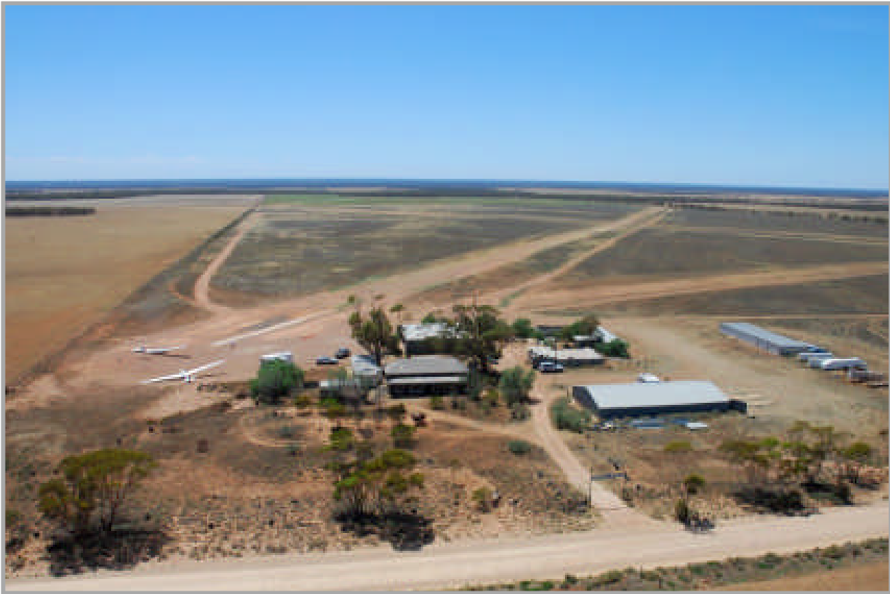
Stonefield Airfield Facilities)
