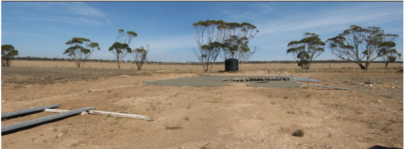
The hangar construction progresses a few more steps...
