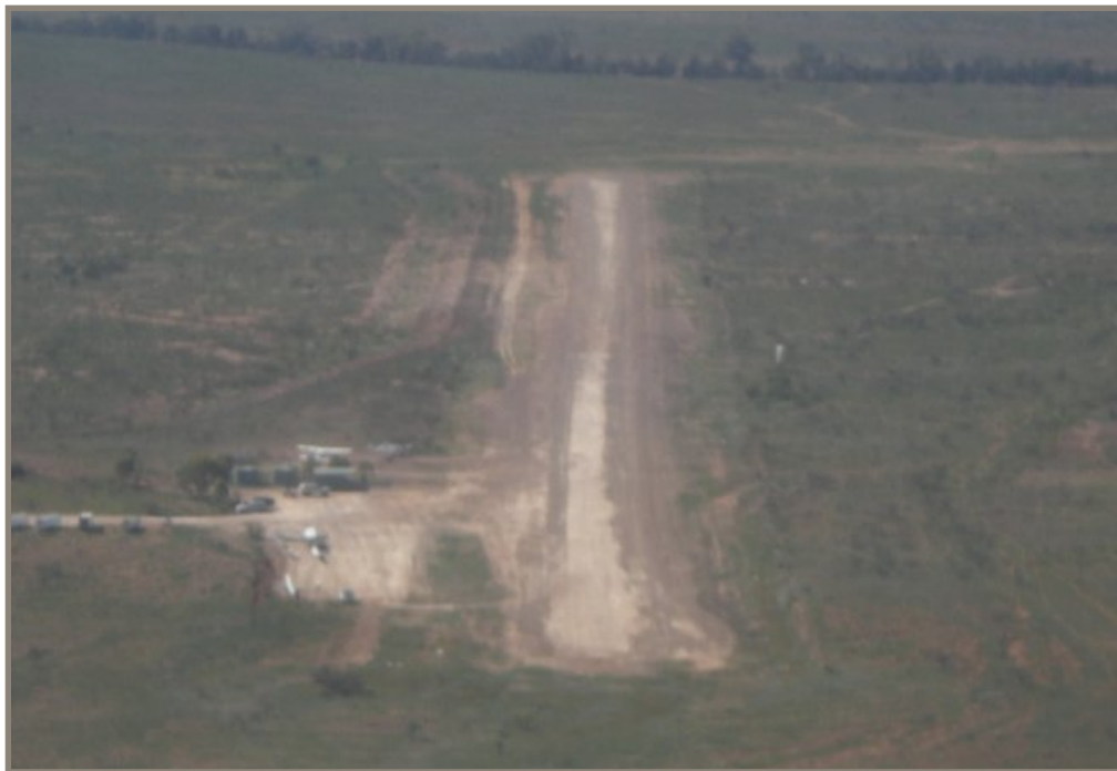
The approach to RWY 03 at Rawnsley Park. The glider tie-down and rigging area can be seen on the lower left. (Photo C. Conway)
