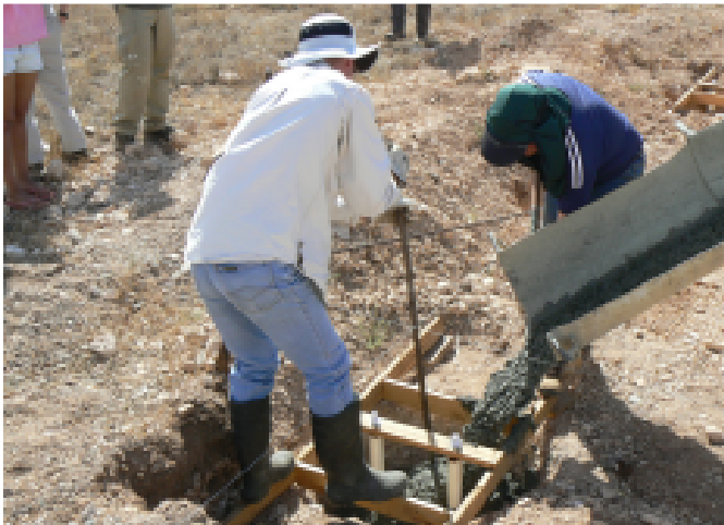
Left: During the pour - note the precision shovel work. Right: After all the dust had settled - 14 concrete filled holes! Photos: D. Medlow
